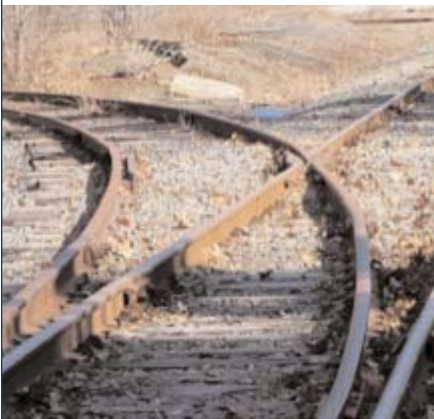
In addition to rail and tie replacement, 15 turnouts will be replaced by the Project.
