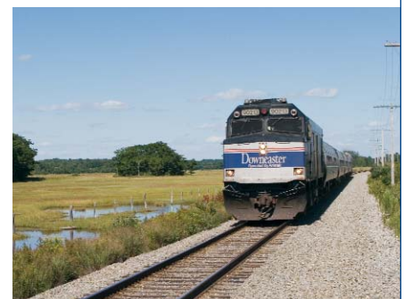
The improvements will result in significantly improved track conditions which will safely and comfortably support the operation of Downeaster passenger trains.
