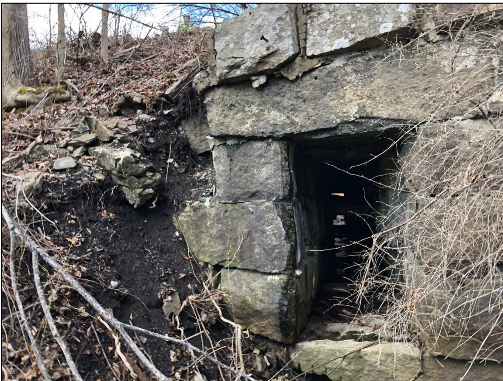
Photo #4: Elevation of Stone Box Culvert Outlet
