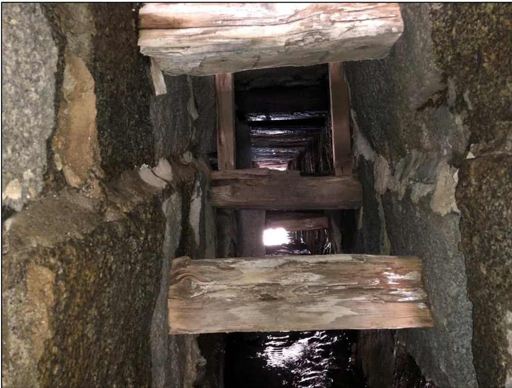
Photo #6: Timber Bracing in Culvert for Approximately 10' From Outlet
