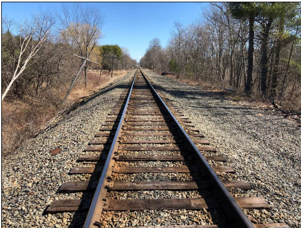
Photo #2: Looking East Towards Portland
