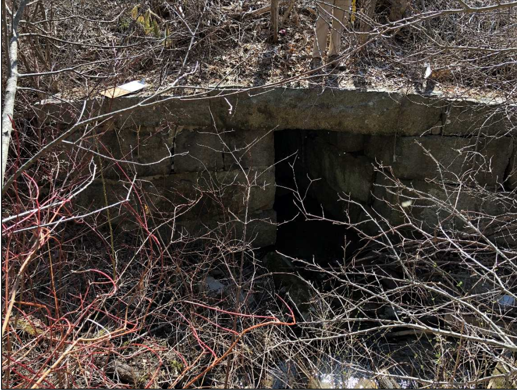
Photo #3: Elevation of Stone Box Culvert Inlet
