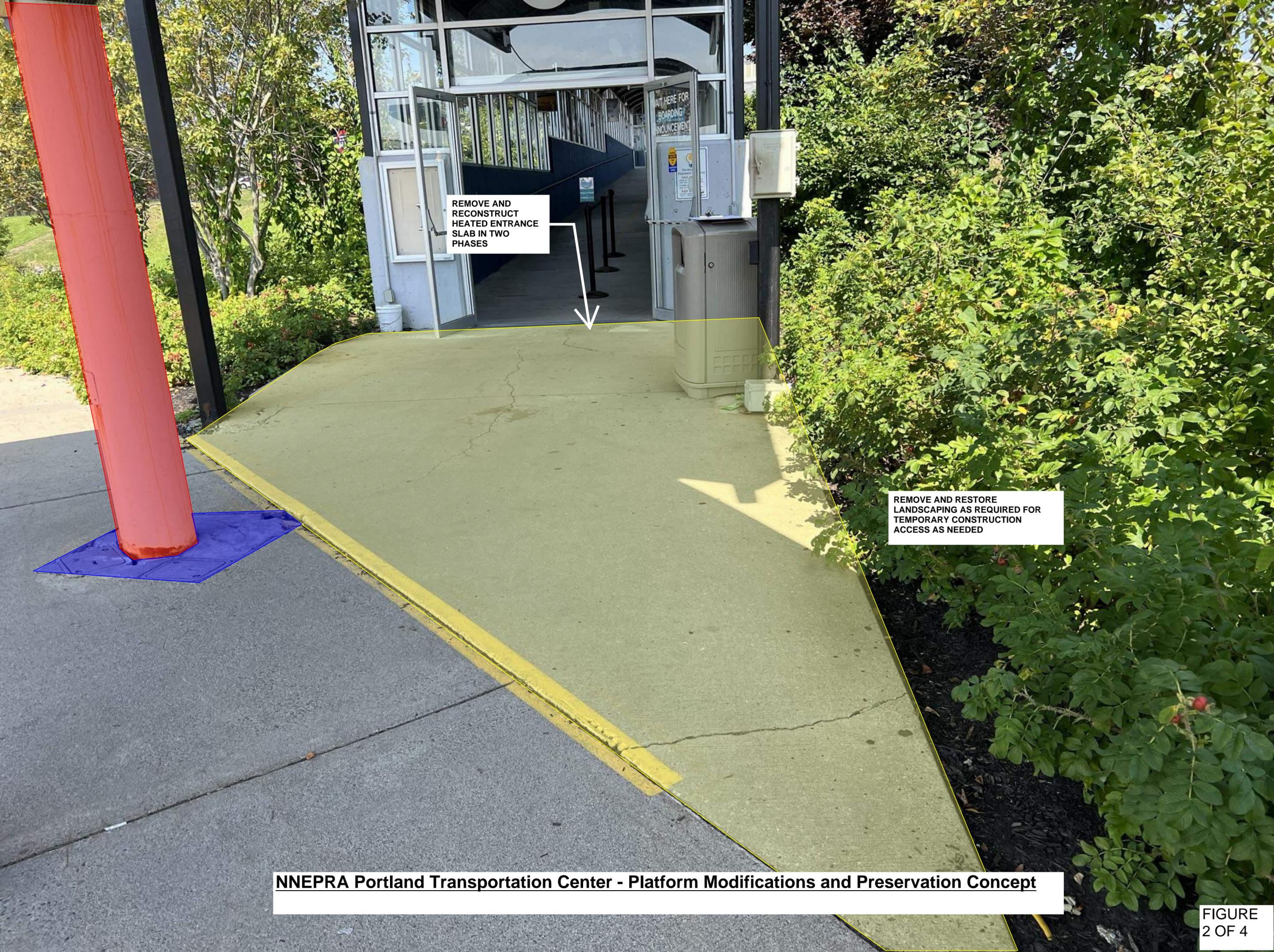
REMOVE AND RECONSTRUCT HEATED ENTRANCE SLAB IN TWO PHASES
